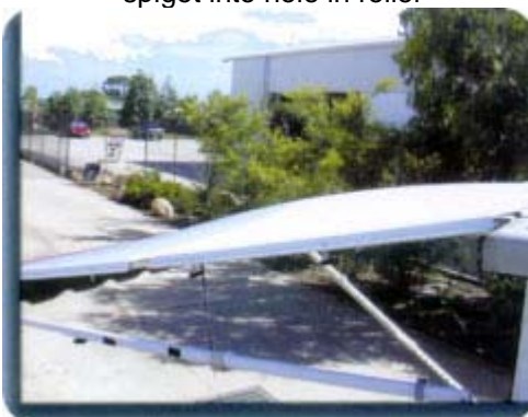
Shows curved roof rafter in position
