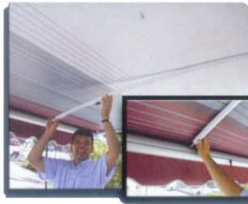
Extend out front telescopic section and fit spigot into hole in roller
