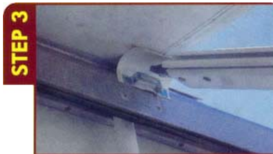
STEP 3 Attach the pole and hook to the wall bracket
